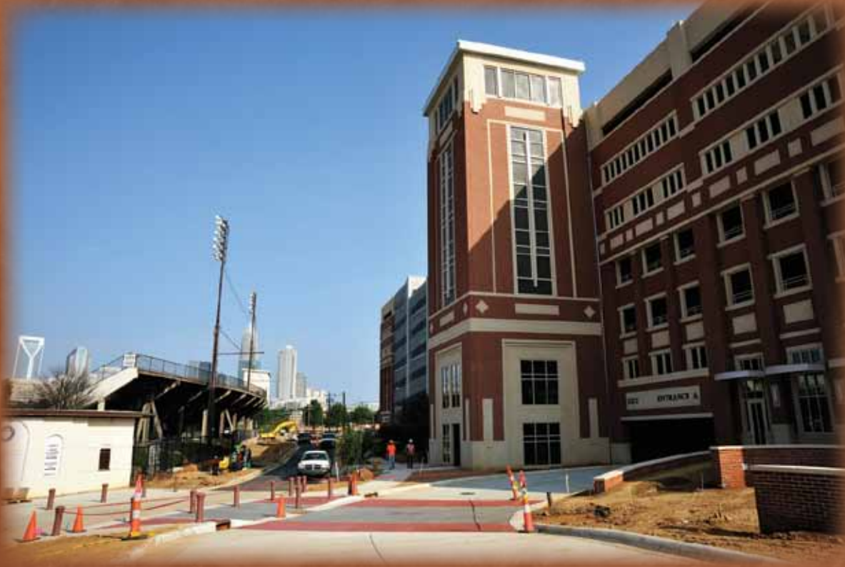
New Central Piedmont Community College Student Parking Deck
