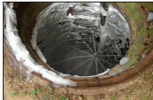
Tree Root Control Program: manhole being treated
