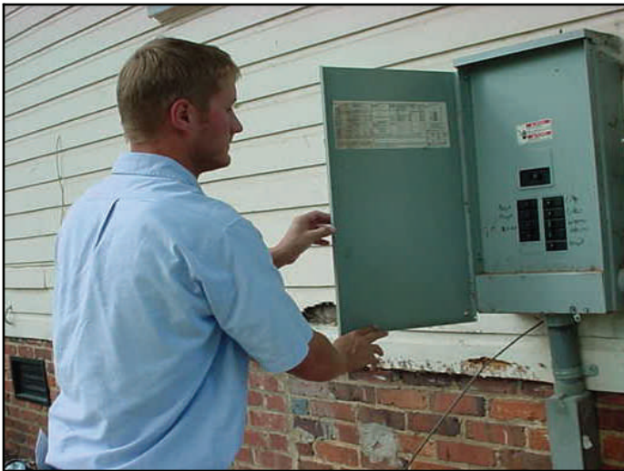
Neighborhood Development Code Enforcement Inspector inspecting a housing code violation.
