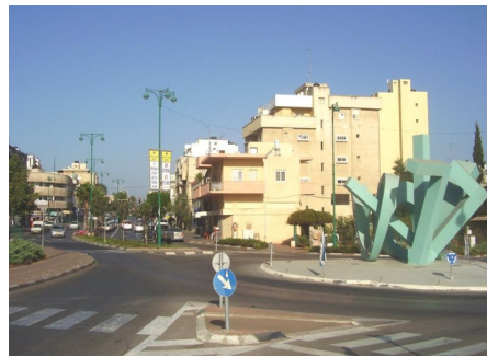
The Tisha (nine) circle, and HaNasi Weitzman street Courtesy: Rck Pelleg
