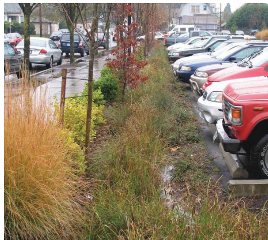
On-site stormwater management at surface parking lots and along streets will reduce runoff while beautifying the environment.
