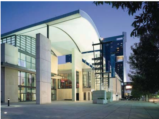
The Charlotte Convention Center should be expanded in ways that augment the facilities while creating attractive, walkable ground-floor environments.
