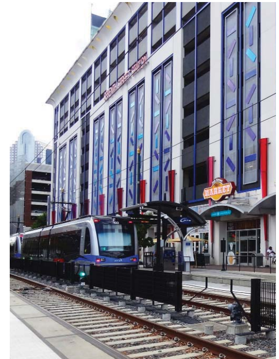
Parking structures should be retrofitted when possible to incorporate elements such as public art and ground-floor retail, similar to those at the 7th Street Station parking deck.
