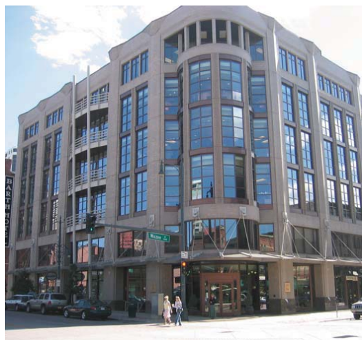
The Hal Marshall site should incorporate nicely-articulated buildings and active ground-floor uses.
