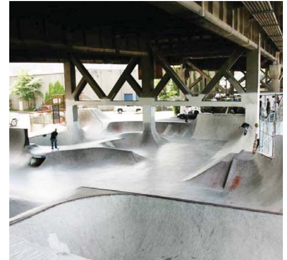
Freeway underpasses can incorporate recreation uses, such as this skate park in Portland, Oregon, to create a sense of activity and “eyes on the street.”
