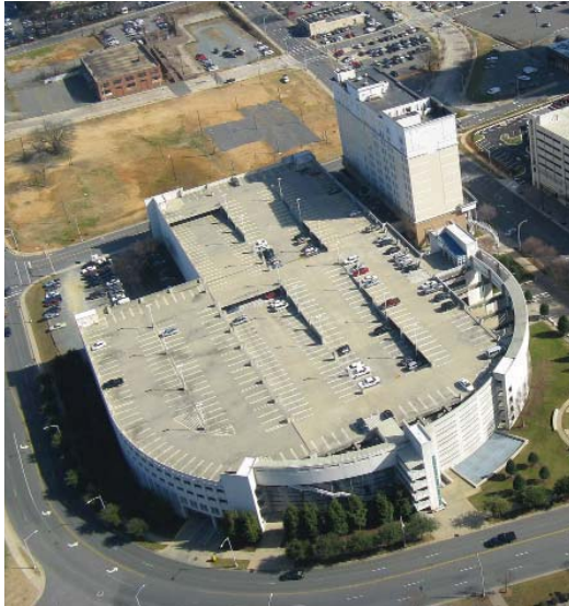
Existing parking structures in Uptown have multiple inactive edges, are often adjacent to other parking facilities and detract from the overall urban fabric.
