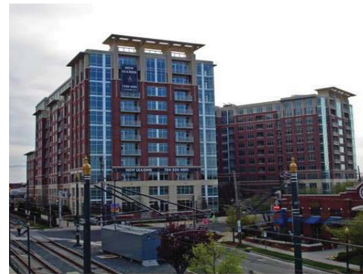
New mixed-use development characterizes several parts of the South End Focus Area.
