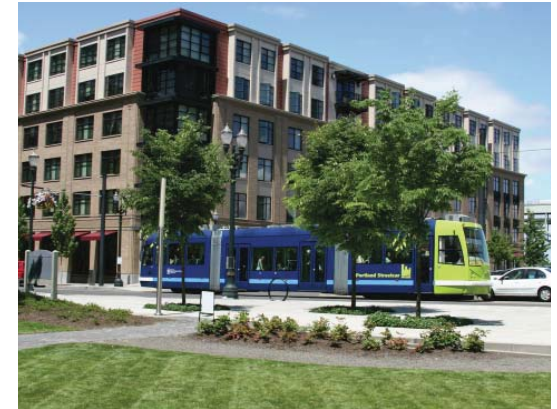
Implementing existing plans for streetcar on West Trade Street will help to link existing destinations and catalyze private development along the corridor.
