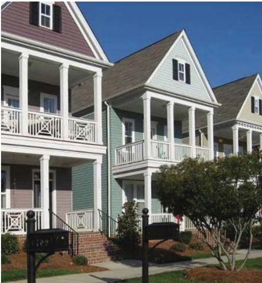
First Ward Place is a Hope VI mixed-income housing project with two- and three-story garden apartments.
