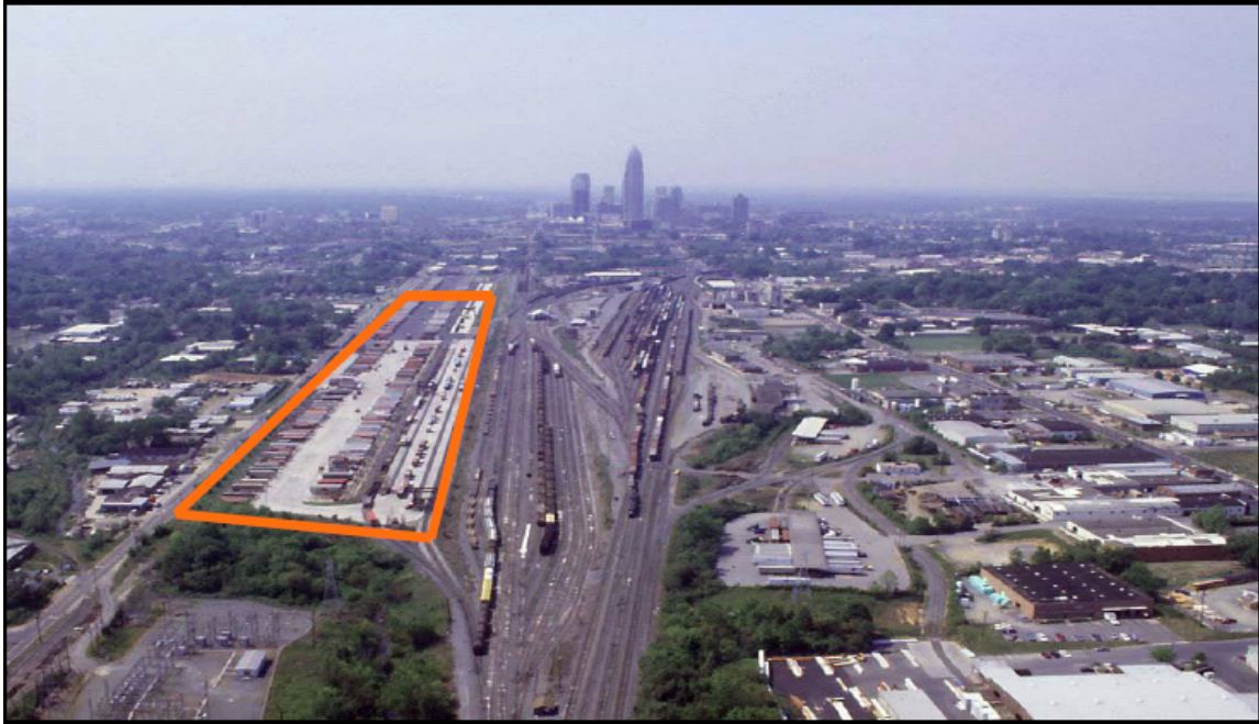
Figure 3-13: Existing Norfolk Southern Intermodal Yard
