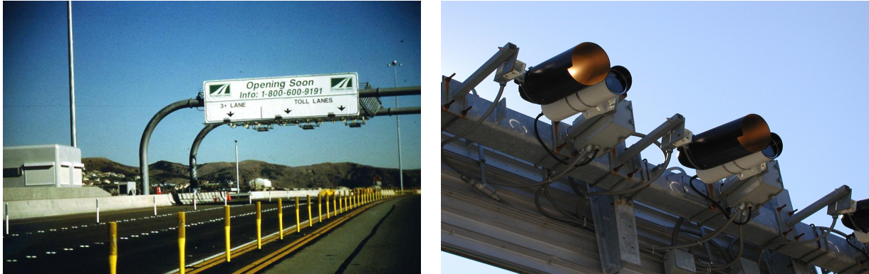
Figure 1-8: Electronic Toll Technology Applied to Managed Lanes
