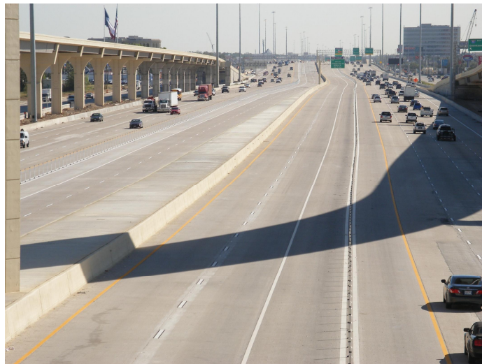
Figure 1-5: Katy Freeway Express Toll Lanes
