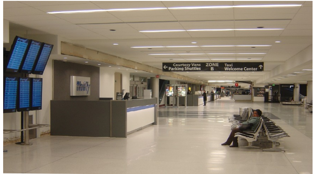
Arrivals/Baggage Claim Area with terrazzo flooring, digital monitors, new ceiling panels, energy-efficient lighting, and counter upgrades
